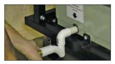
➤ Unwrap and install the thermostat. Make a small opening in the bottom of the upper duct opening and pass the thermostat through, along with 50' of cable.
