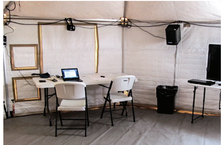
Air Purifier installed in a 1935 Shelter System
