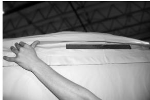
Make sure the corners of the vented end cover completely cover the junction of the wall and roof panels.
