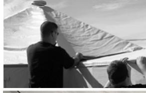
j. When connecting roof panels, make sure the fastening strips seal completely in the corners where the Hygiene Center meets the shelter.
