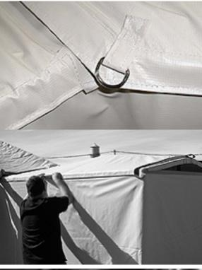
k. Working out from the shelter, connect the Hygiene Center roof and wall panels.
