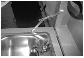
f. Position the assembled sink against the wall on the shower side of the Hygiene Center.
