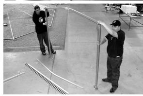
i. Lock the leg bars into place, using their captive locking pins.
