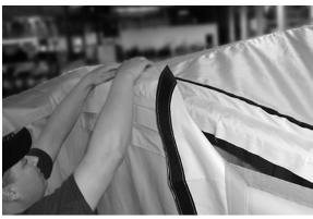
I. Attach the vented end cover panel to the roof panel. Start at the center seam and work your way out to the ends.
