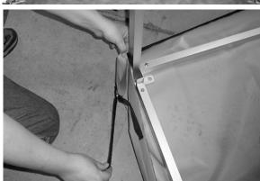
p. When properly fitted, the floor panel should wrap around the frame to a uniform height of 6"
