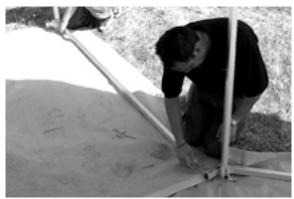
m. Connect the arched ridge bar between the shelter arch bar and end frame assembly. Again, keep the eave bar supported at all times during installation.
