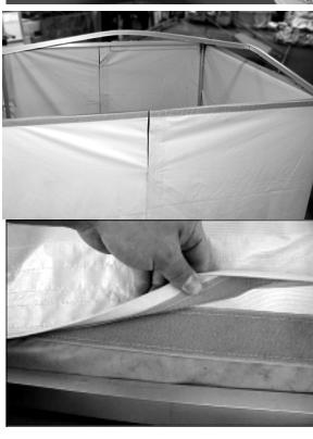
d. Inside the Hygiene Center, attach the floor to the weather flap running along the base of each wall panel.
