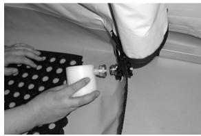
e. Orient the strainer so the open end is pressed against the stall floor.
