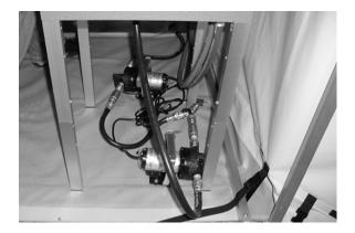
c. Each DPP-550 sump pump ships with an electrical switchbox. Hang the switchboxes from the eave bar above the pumps. Plug each pump into its switchbox, and connect the switchboxes to a 115VAC power supply.
