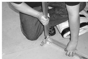
k. Connect two straight eave bars (one from the Hygiene Center kit and one removed in step **c**) between the lower ends of the shelter arch bar and the end frame assembly. The black fastening strips should face out.
