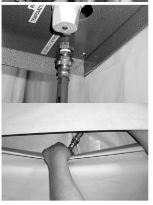
e. Coil the remaining hoses and tuck them into the gap between the shower stall and the Hygiene Center wall.
