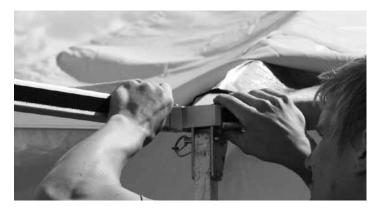
Connect the arched ridge bar (from the Entryway Kit) to the center position on both the shelter and the End Frame Assembly.
