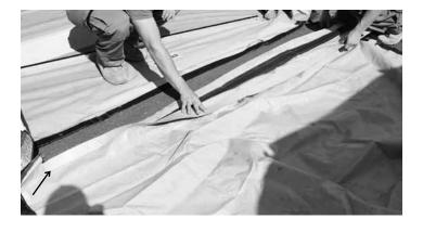
Align the center indicating arrow with the indicating arrow on the shelter floor.
