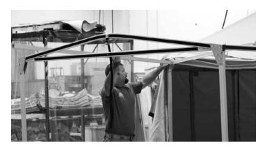
Install the entryway base bar (with labels) between the legs of the End Frame Assembly.
