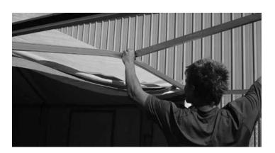
With one person supporting the end frame assembly disconnect and remove two entryway eave bars.
