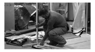
Install the 90 degree angle base bar assemblies between the shelter and the End Frame Assembly.
