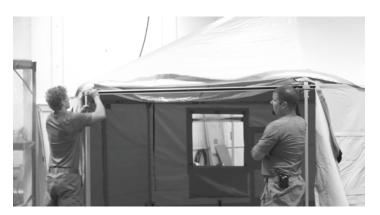
Install the arched eave bar with the hook & loop fastener facing inside the shelter.
