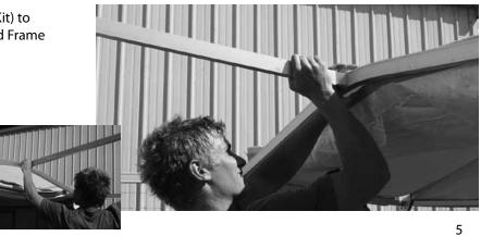
Connect the remaining eave bar (from the Entryway Kit) to the remaining corner block on the shelter and End Frame Assembly (hook & loop fastener facing outside of shelter.)
