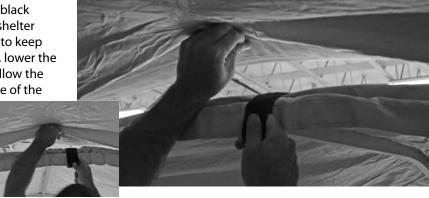
First, determine the insulation wall type based on the entryway location (door connection or side connection). Attach the insulation wall panels by starting at the door frame. Attach the hook & loop fastener to the corner of the door frame and the top of the eave bar and secure the fastener down the length of the door frame.
