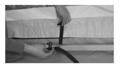
Peel back wall section exposing the shelter frame legs and remove door if necessary.
