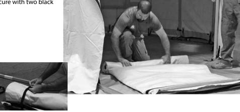
Remove entryway wall panels and layout on shelter floor for folding.
