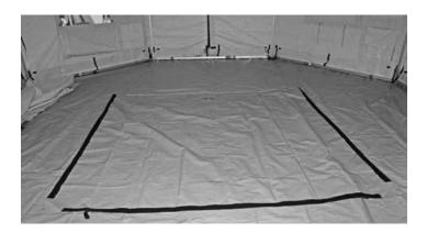
Fold each side of entryway floor to the center line two times.
