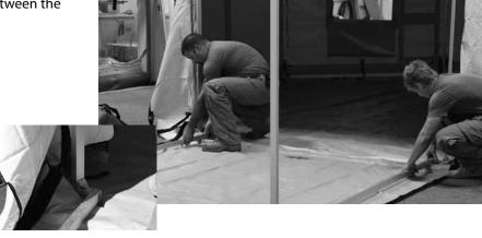
Install the Door Assembly on the End Frame Assembly making sure that it aligns with the center mark on the frame. Also ensure that the Door Assembly in securely supported by both the eave and base bars.
