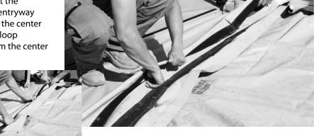
Connect the two square tabs from the entryway floor to the two square tabs on the shelter floor as shown.
