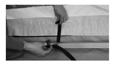
To attach the end cap, start at the center seam and work toward the ends. After the end cover has been attached to the roof panel, attach the bottom of the vent to the wall panel.
