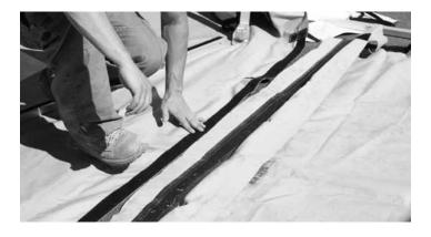
Fold the shelter floor's hook & loop fastener so that the fastening strip is facing down and connect to the entryway floor's hook & loop fastening strip. Make sure that the center indicating arrows are aligned and that the hook & loop fastening strips are straight and aligned. Work from the center out to both sides of the connection.
